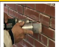
Fast, Precise, Brick Mortar Removal
